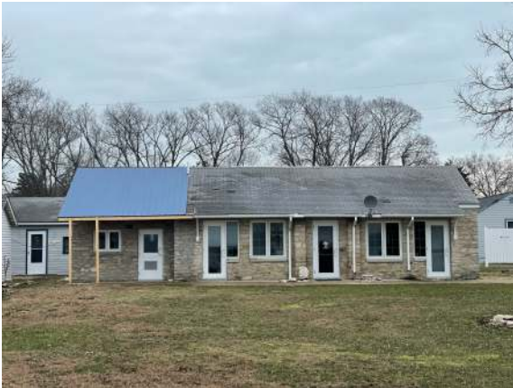
New metal roof over laundry room
